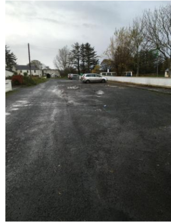
Parking markings should be re-painted outside the school
