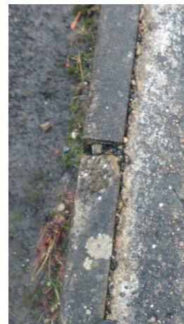
Some pavements cracked
